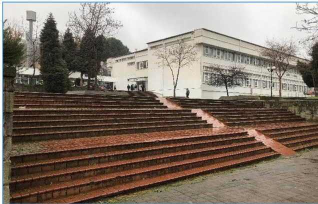
Fig. 15. Narrow and steeply sloping ramps
