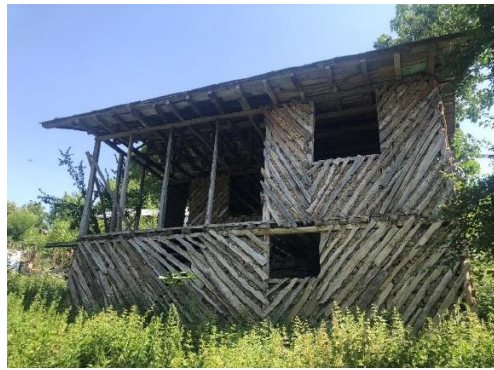
Fig. 4. A Half-Built House with a Zegali Structure
