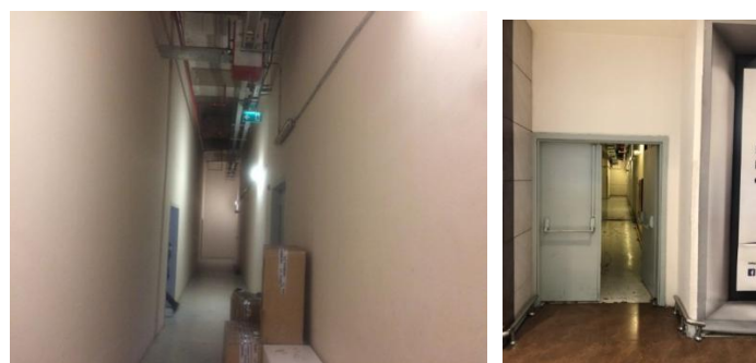
Fig. 2. Emergency exit doors of fire escape routes
