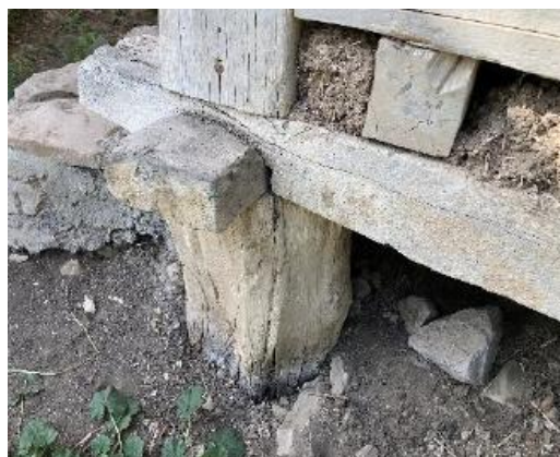
Fig. 2. Pakouné foundation and the way of its connection to Bone Nal
