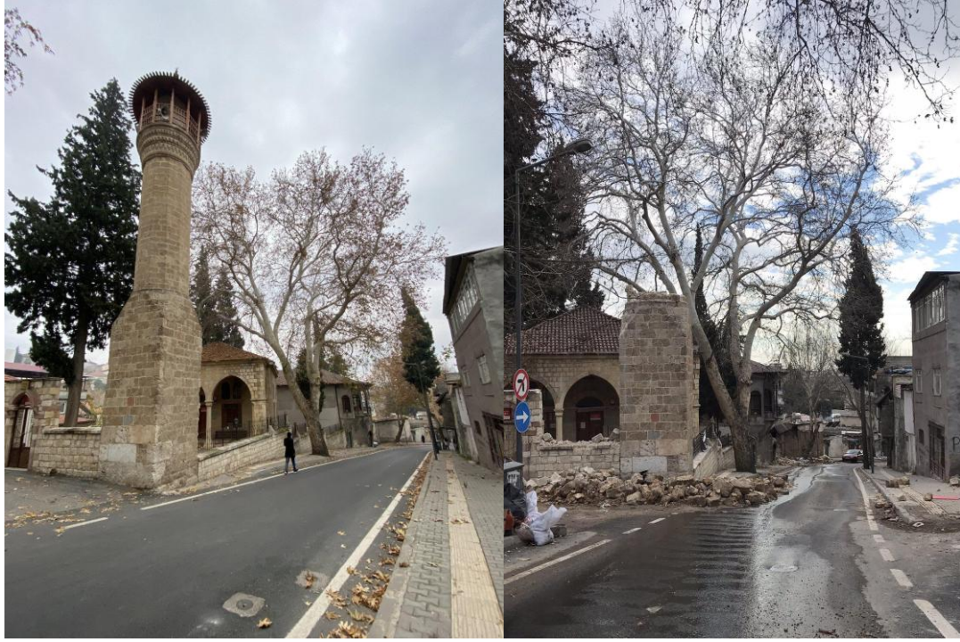
Fig. 2. Damage to the minaret of Çukuroba Mosque, before (Z.Aytemiz) and after (F.AI) earthquake
