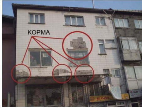
Fig. 2. Coatings falling off the facade of the building due to heat change (Güzelçoban Mayuk, 2007)
