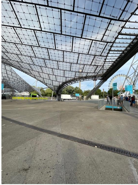
Fig. 4. The view of the end cables coming from the end of the cantilevered roof to the ground (photo by B.Orbay and Y.K. Aktuglu, 09.08.2024)
