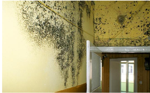
Fig. 5. Fungus and mold formation in the building (Interior, 2023)
