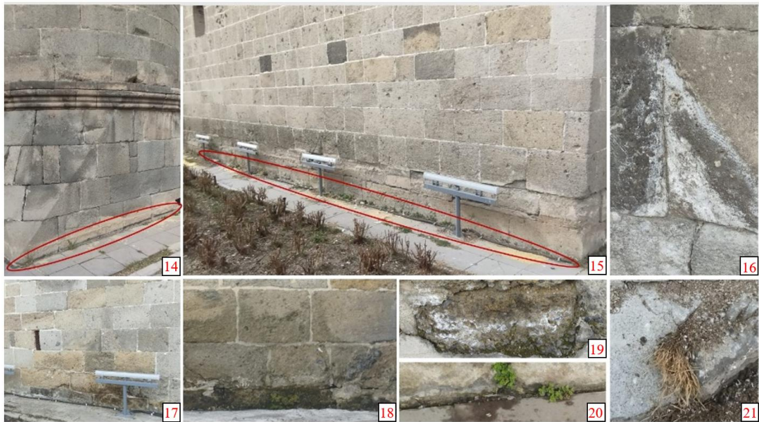
Fig. 11. Erosion, Salt Crystallization, and Biological Colonization on the Stone Material of the Yakutiye Medrese (Author Archive, 2025)
