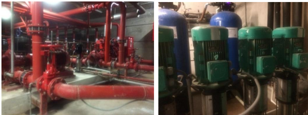
Fig. 6. Fire Pumps and booster systems
