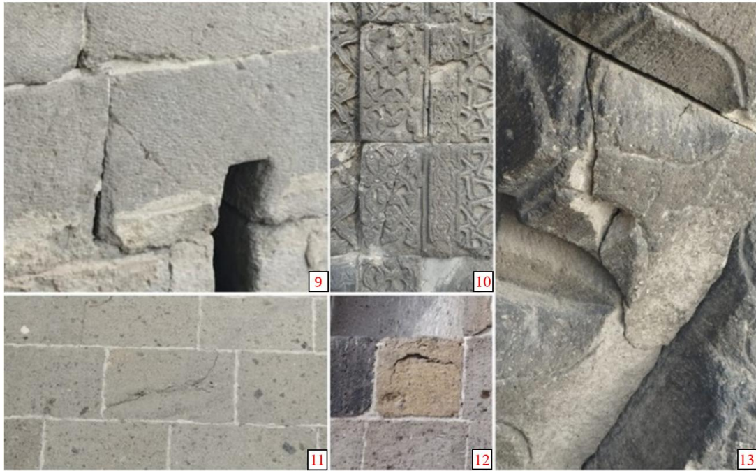
Fig. 10. Cracking and fracture in the Stone Material of the Yakutiye Medrese (Author Archive, 2025)
