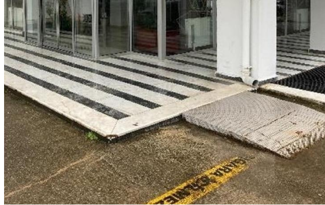
Fig. 9. A ramp without handrail
