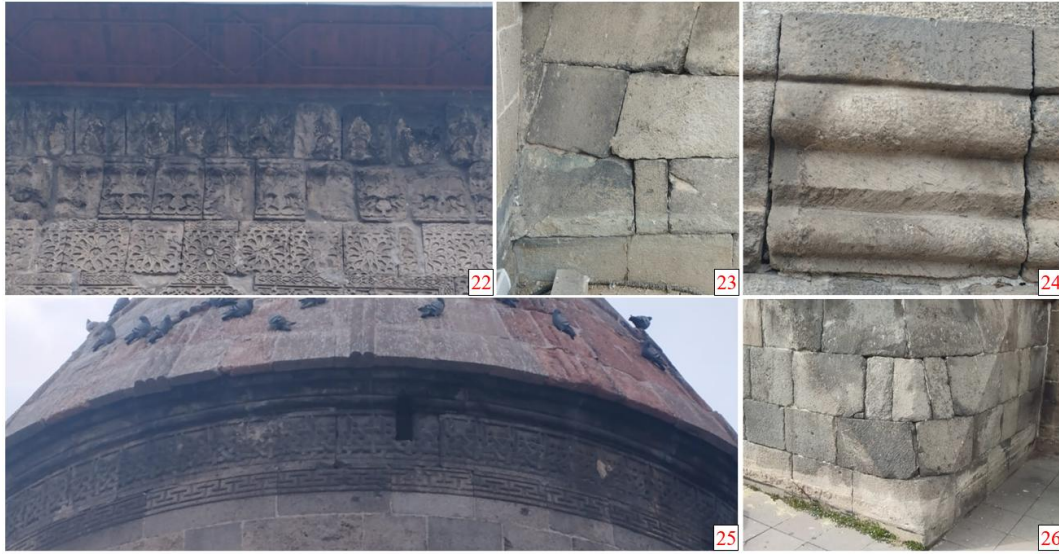
Fig. 14. Joint deterioration and Soiling on the Stone Material of the Yakutiye Medrese (Author Archive, 2025)
