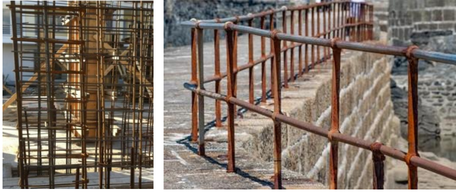
Fig. 4. Corroded column reinforcement (left), corroded railing (right) (Dal & Yılmaz, 2015; Peter, 2025)
