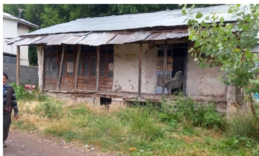
Fig. 6.Tow-sided roof with tin
