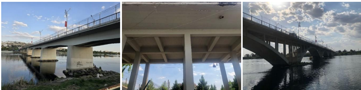
Fig. 2. View of the bridge's reinforced concrete beam section from the west bank; the reinforced concrete beam system supporting the deck slab; view of the bridge's reinforced concrete arch section from the east bank (Personal Photography Archive of Author, 2025)
