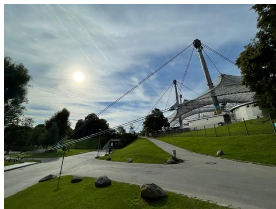
Fig. 3. The view of the cables coming from masts and roof to the ground (photo by B.Orbay and Y.K. Aktuglu, 09.08.2024)
