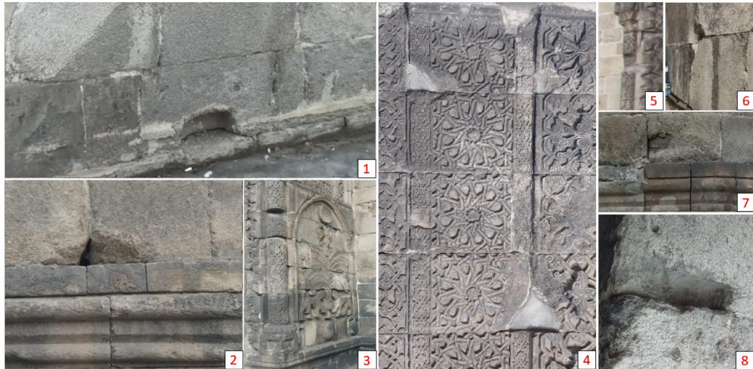
Fig. 9. Loss of Pieces in the Stone Material of the Yakutiye Medrese (Author Archive, 2025)
