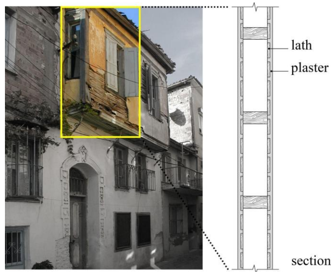
Fig. 2. An example of the “bağdadi” construction technique in Ayvalık traditional houses
