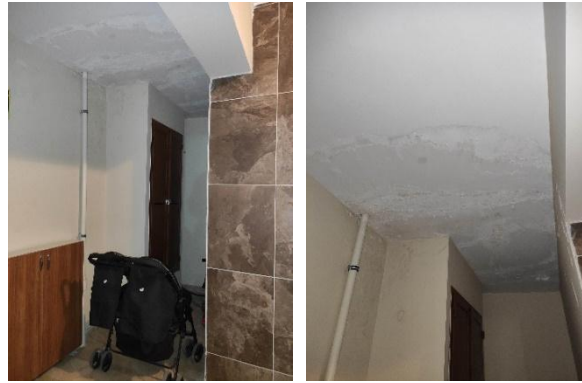
Fig. 3. Swelling and flaking seen in the ceiling paint as a result of the effect of water and humidity in the building (Özdoğan, 2023)
